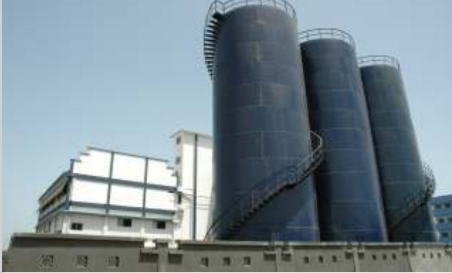
An Industrial unit in SURSEZ
